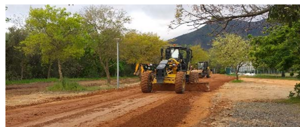
Photo: Civil contractor filling eroded gravel roads in the Stellenbosch Mountain.
