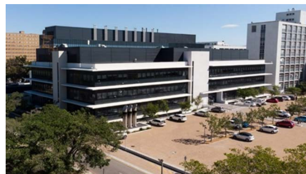
Photo: BMRI building at Tygerberg
