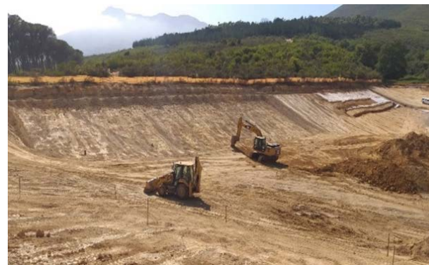
Photo: Ertjieskloof dam construction
